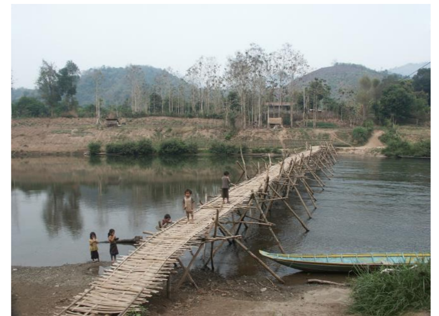
A temporary river bridge
